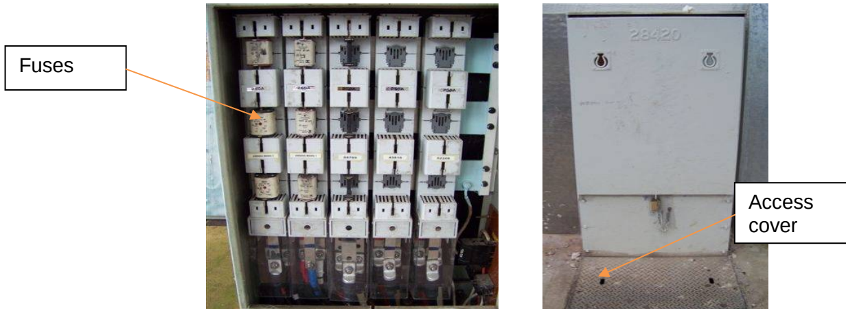
Figure 13: Typical DFP with cover off and cover replaced (internal switchgear may vary)
