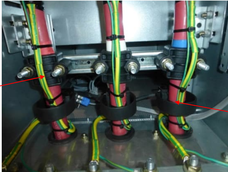
Fig. 3 Installed black colour CTs (pre-February 2020)
