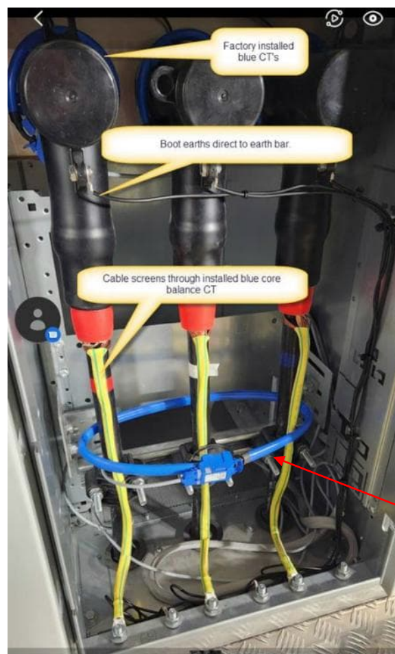
Fig. 4 Installed blue colour CTs (post-February 2020)
